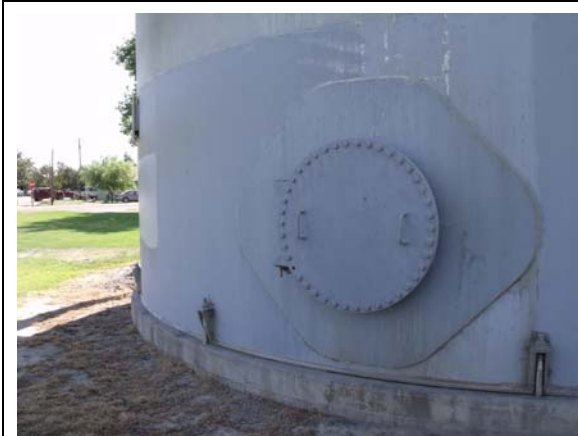
800,000 gal. Welded Steel Reservoir
