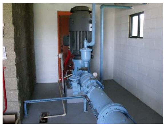
Well No. 4 – Motor and Piping
