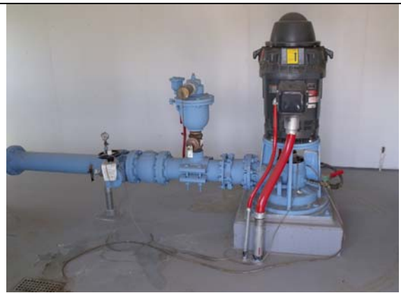
Well No. 5 – Motor and Piping
