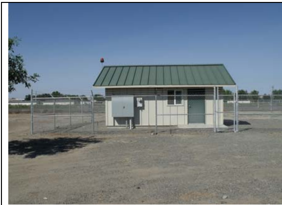
500 gpm Well No. 5 Well House
