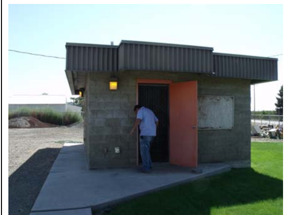
200 gpm Well No. 4 Well House
