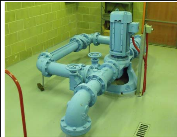
BPB Fire Pump and Bypass
